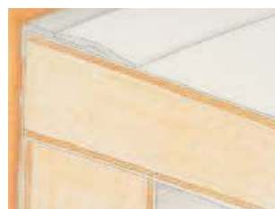
Bonding of a roof-element with Körapur 140
