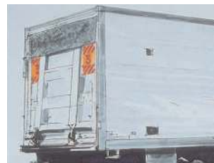
Covering the hydraulic platform with Körapox BS 90
